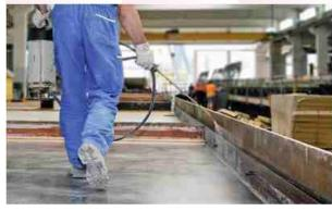
predetermined sizes. The physical characteristic of this mineral originated powder mix is to enhance the surface strength of concrete floors and also to impart abrasion resistance against traffic movement.
