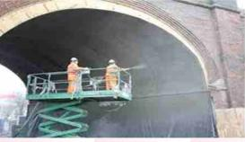
VITCON 9013 AFS is a high performance, alkali free powder accelerator for dry shotcrete mix. This product is formulated to increase the rate of hardening of cement and concrete mixes and this can be controlled by varying the dosage to the sprayed concrete
